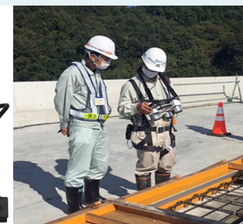
Inspecting rebar arrangement
